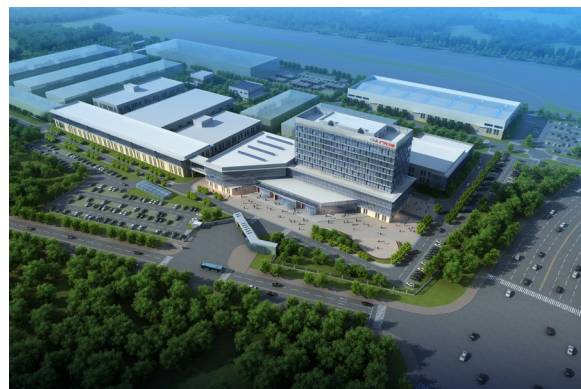
GAC Mitsubishi's R&D Center
